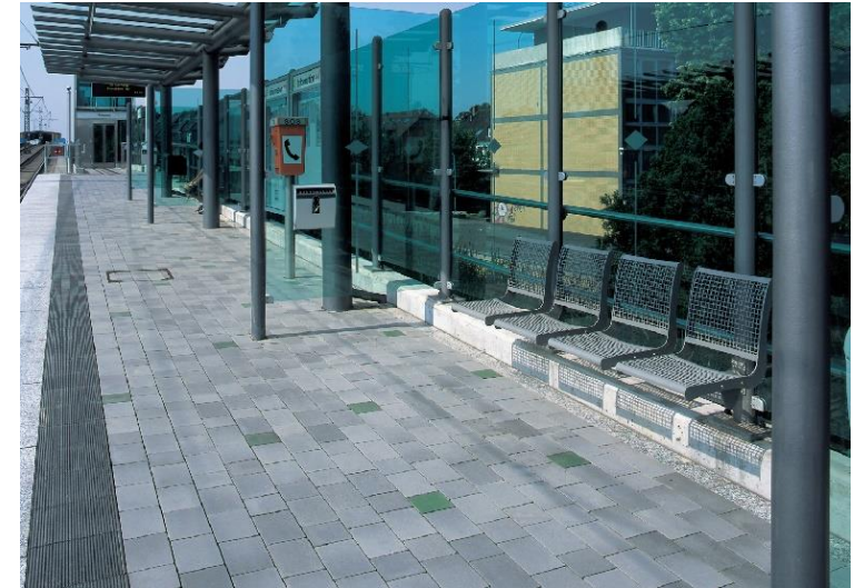
After cleaning, pavers look brand new.
