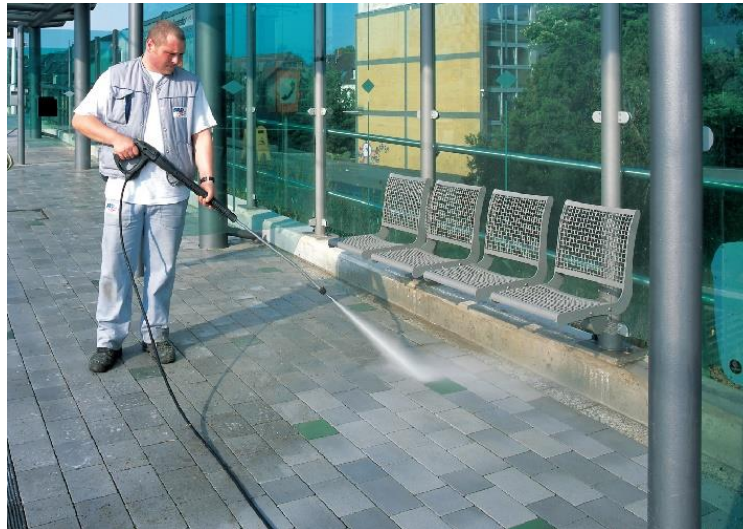
Pavers are simply power washed with soap and water.
