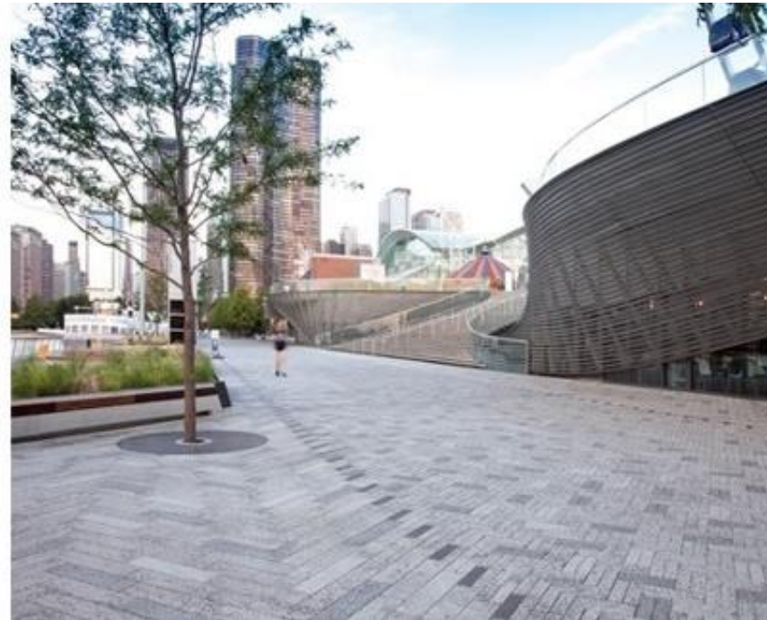
Custom color and shapes created for Navy Pier, with 30% recycled content (Chicago, IL)
